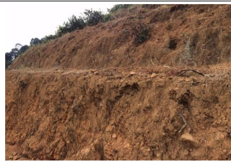
Photograph 6° During the onsite audit, it is still found landslide beside the boundary of the tea plantation and also along the public road.
