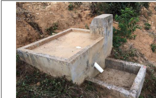
Photograph 5° There is no eyewash facility in the areas where agrochemicals are mixed and distributed.
